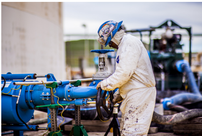
Figure 1. Lining up speciality equipment for non-entry tank cleaning.
