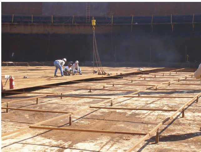
Figure 3. Installation of a new external floating roof (EFR) in an existing storage tank.
