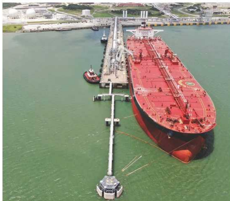
Planned modifications by Matrix to the finger pier at the Moda Ingleside Energy Center will allow for the simultaneous loading of an additional 40,000 barrels per hour from each of its two berths.
