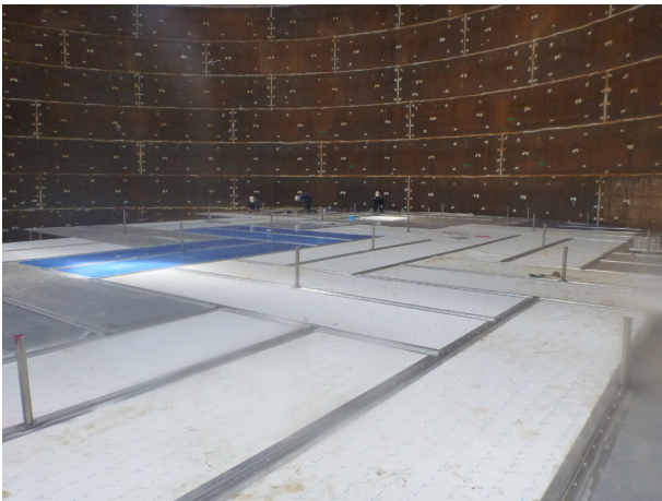
Figure 2. Bolted-style aluminium floating roofs.
