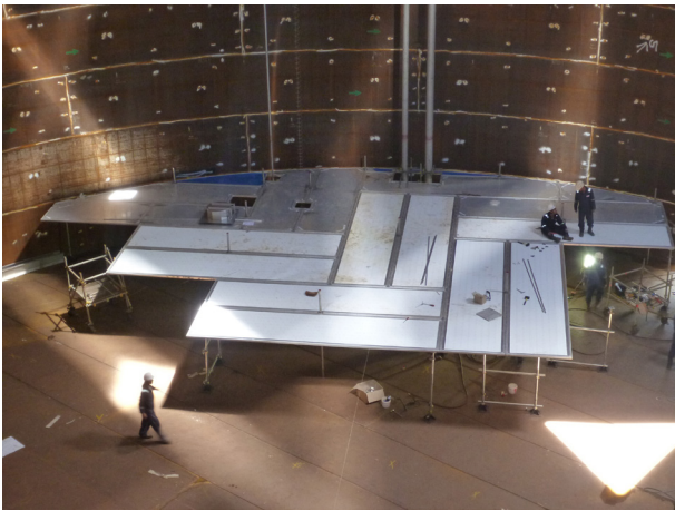
Figure 1. The modular nature of a bolted full-contact aluminium internal floating roof makes replacing panels much easier in the event of a needed repair.
