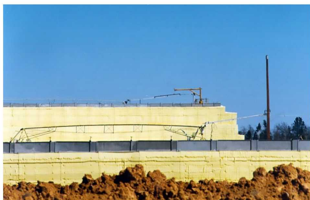
Figure 5. Two large sulfur storage blocks with forms and pouring arms.
