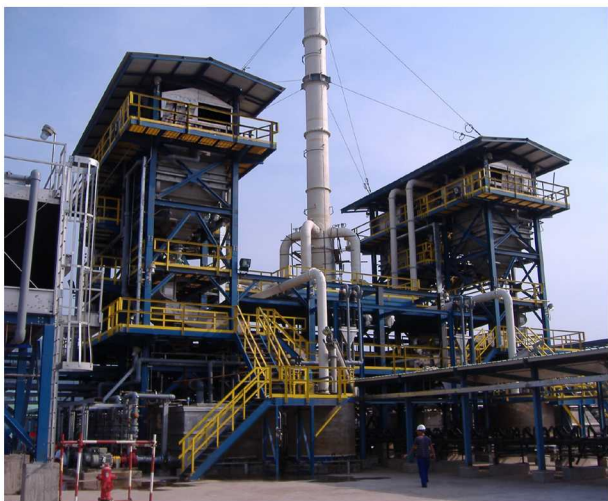
Figure 1. Priller units showing space-efficient tower design.
